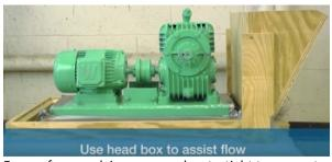
Ensure formwork is secure and watertight to prevent movement and leaking during the placing and curing of the grout. The area should be free of excessive vibration. Shut down adjacent machinery until the grout has hardened. In hot weather, base plates and foundations must be shaded from direct sunlight. Bags and buckets of grout should be stored in the shade prior to use. In cold weather, the temperature of base plates and foundations should be raised to over +10°C
