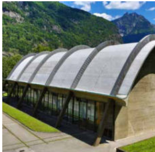
Project year: 1967 | Nuova Biaschina Hydroelectric Plant, Personico, Switzerland | Sarnafil® G 410-12
