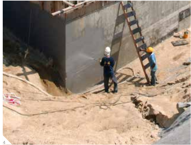
4 Liquid applied reactive membranes (PUR/PUA)
