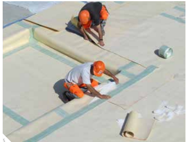
5 Fully bonded sheet membranes
