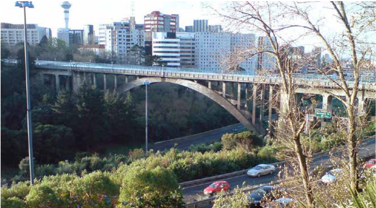
Grafton Bridge, Auckland, New Zealand
